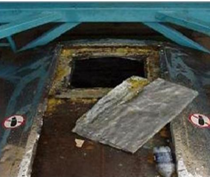
Roof of Container (tank container)
